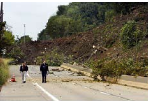
Landslide in Kilbuck, PA (2006). Photo courtesy of the Pittsburgh Post-Gazette.
